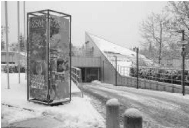
Figure 4. Main entrance of ZSM downward to underground (photo: M. Müller, in wintertime).
