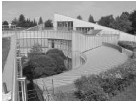
Figure 6. View over one of the two circular courtyards, at the lower right the library; behind the triangular top of lecture hall and solar panels.
